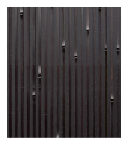
Sumushiko is a latticework made from 5 mm-thin flat-split bamboo strips, assembled at regular intervals. The uniform spacing creates a refined pattern of light and shadow, lending visual depth and a sense of lightness to interiors. Each strip is precisely and carefully hand-split in-house to ensure consistent width and
